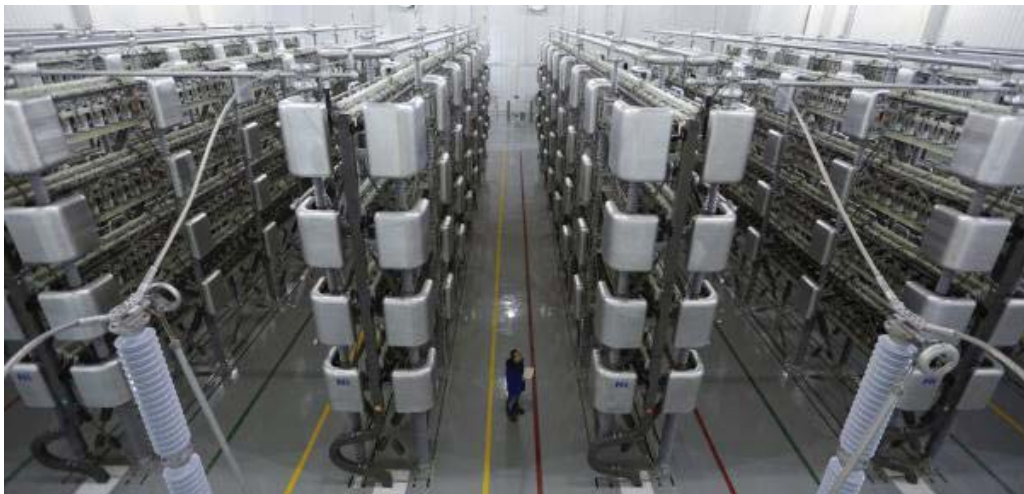
Figure 1 ±160kV/100M VSC-HVDC Converter Valve
