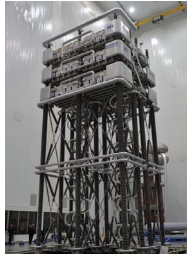
Figure 2 ±535kV/3000M VSC-HVDC Converter Valve
